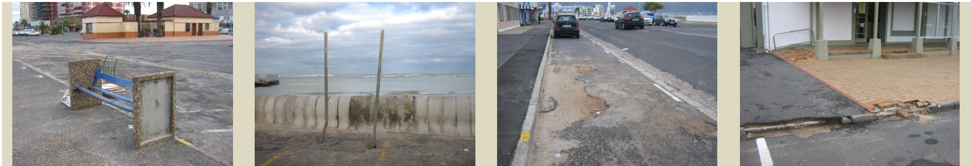
Figure 19 Typical damage to public and road infrastructure in the Strand CBD
