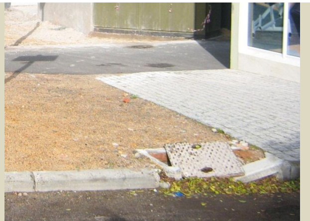
Figure 17 Broken manhole covers on sidewalks
