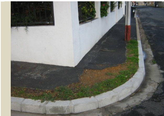
Figure 16 Unmaintained sidewalk surfaces
