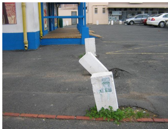
Figure 43 Poorly maintained bollards
