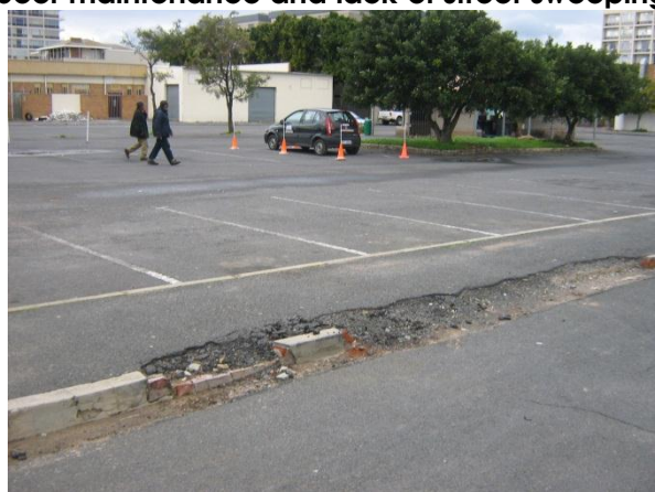
Figure 46 Damage to kerb stones
