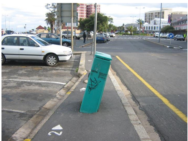
Figure 40 Public infrastructure in a state of disrepair
