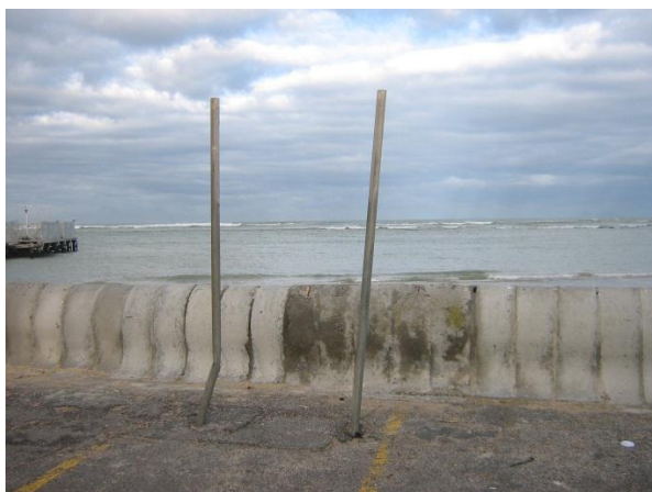
Figure 42 All that is remaining of this public notice sign
