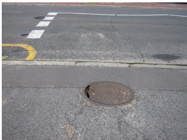
Figure 37 This broken manhole cover makes this sidewalk unsafe
