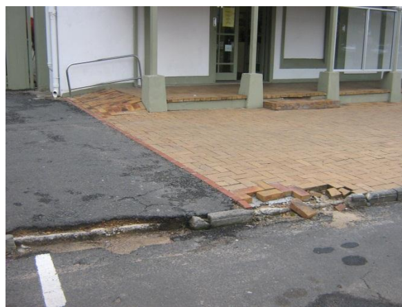
Figure 47 Damaged kerb inlet and kerb stones
