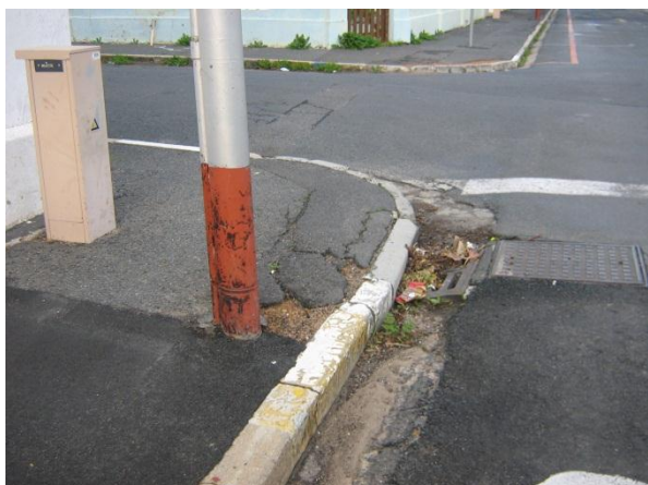
Figure 44 Kerb inlet and drain blocked due to poor maintenance and lack of street sweeping
