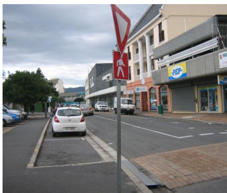
Figure 30 Bent regulatory road sign
