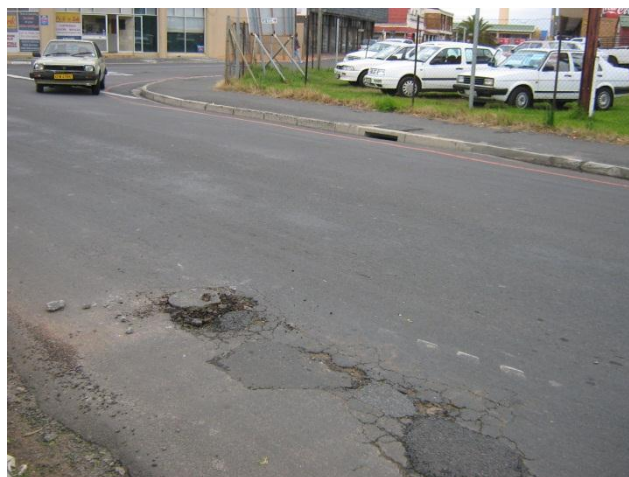
Figure 49 Potholes
