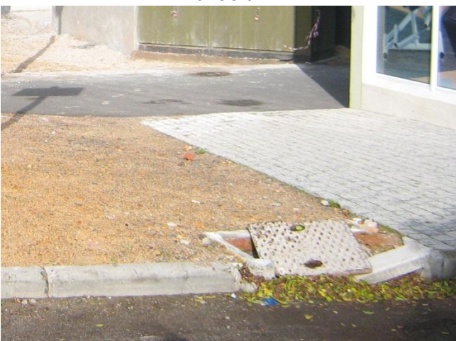
Figure 38 Another storm water manhole without proper cover
