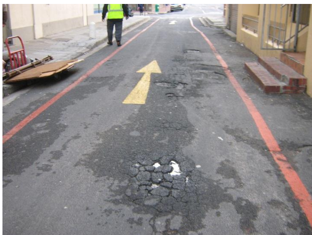
Figure 48 Potholes
