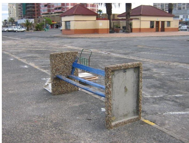
Figure 41 Broken street furniture such as benches that are unsafe to use
