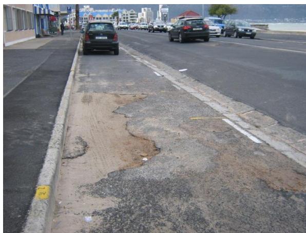
Figure 45 Evidence of poor road surfaces
