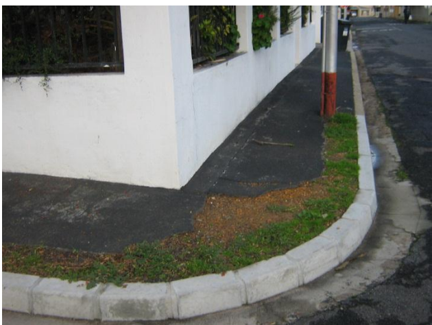
Figure 36 Poor sidewalks in some of the side streets
