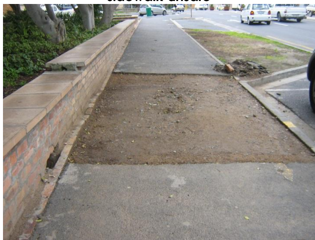
Figure 39 Sidewalk maintenance not completed in the main road
