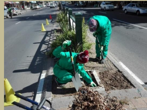
Workers from the Helderberg Night Shelter at work in the Somerset West CBD
