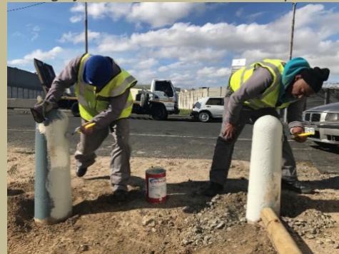
Previously homeless men living at a shelter in Bellville repaints public infrastructure in the Elsies River CID
